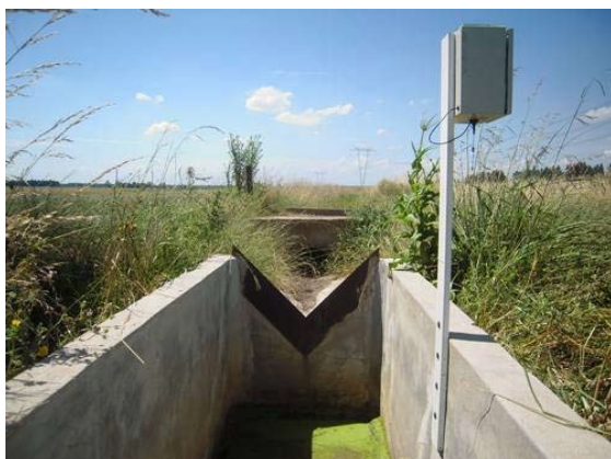
Figura 4-14 Vertedero triangular
